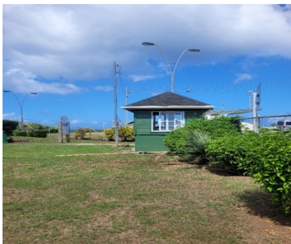
Upgrade to Fort James Security Booth
