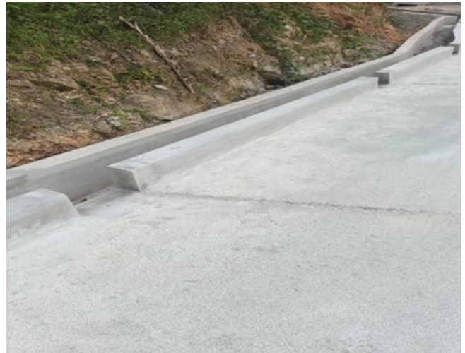
Ongoing works at Gale Agard Road – Bloody Bay
