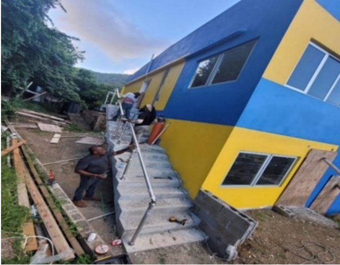
Installation of external stainless-steel handrails
