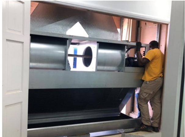
Installation of 25-ton AC Unit
