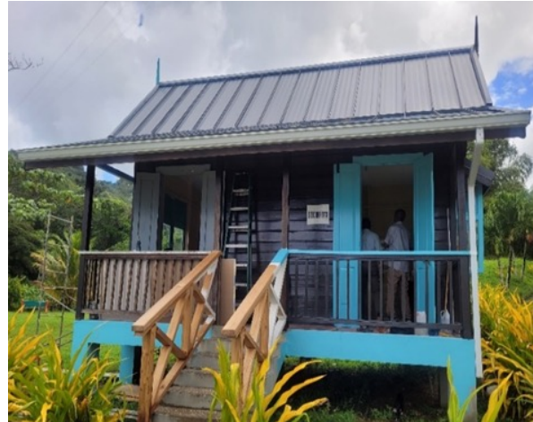
Completed upgrade to Security Booth at Bloody Bay Beach
