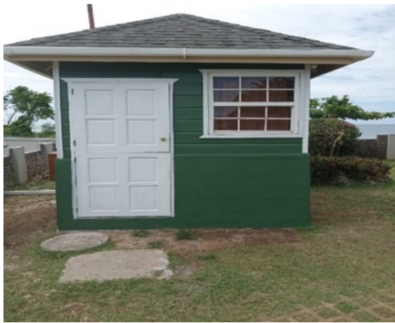
Upgrade to the Security Booth completed
