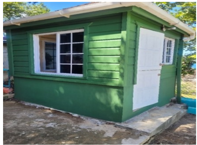
Security Booth at Fort Milford Bennett upgraded
