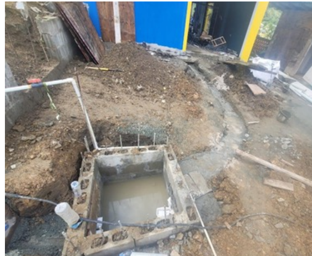
Construction of electrical pull box
