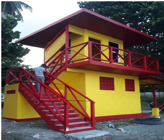
Completed upgrade to the Lifeguard Tower at Speyside Beach Facility
