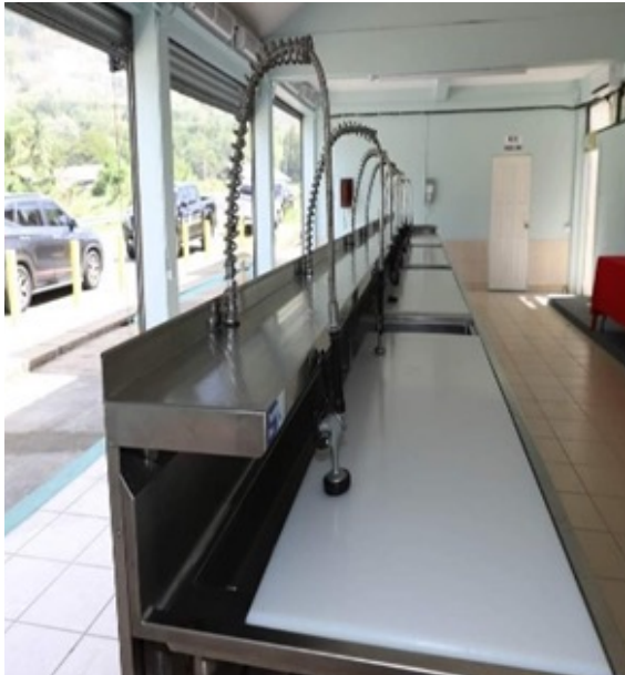
Completed work at Barbados Bay
