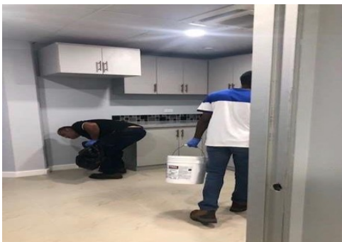
Application of Baits and Chemical for Repairs to Water Pump
