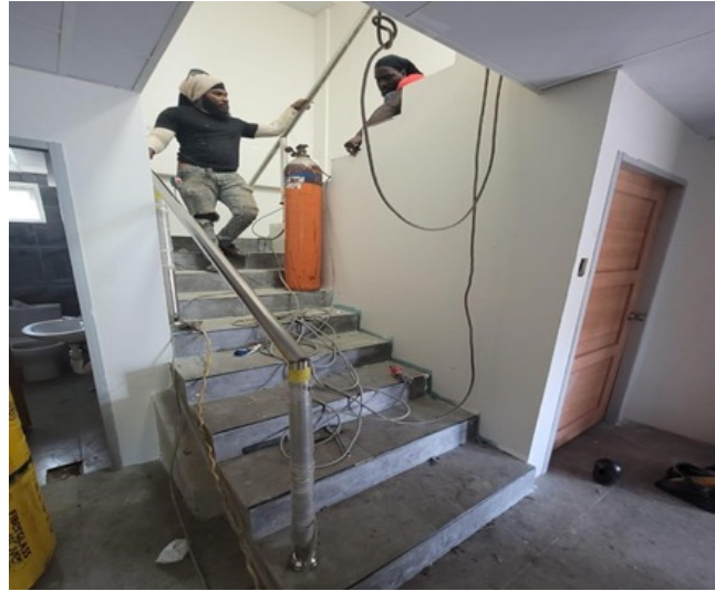
Installation of external stainless-steel handrails
