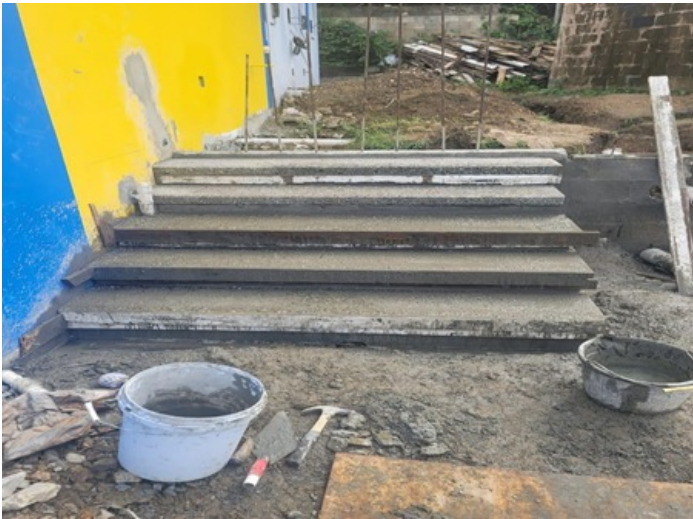
Construction of the external stairs
