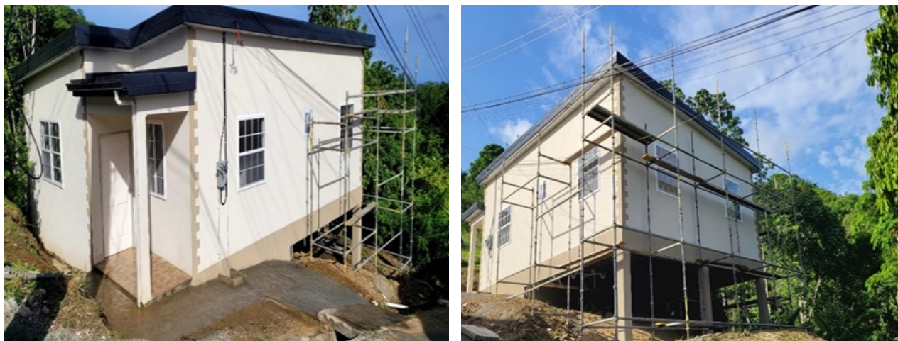
The Home nearing completion under the Social Assistance Housing Programme
