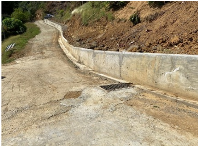
Ongoing works at Big Hole – Goodwood
