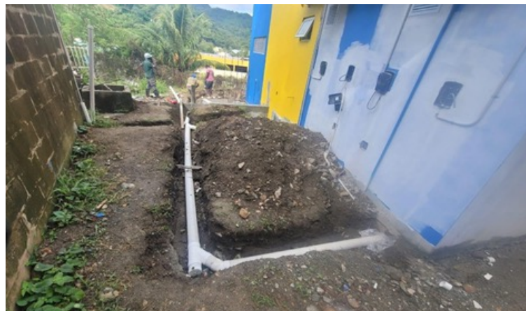
Plumbing works inside of the apron
