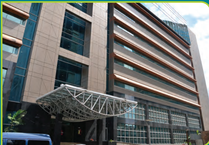
The new Customs House, located at the Government Campus Plaza.
