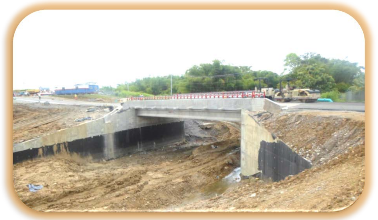
Construction works at B1/3 Calcutta Road No. 2 bridge, Calcutta
