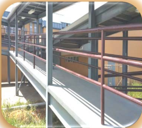
Extension of the roof of the steel ramp
