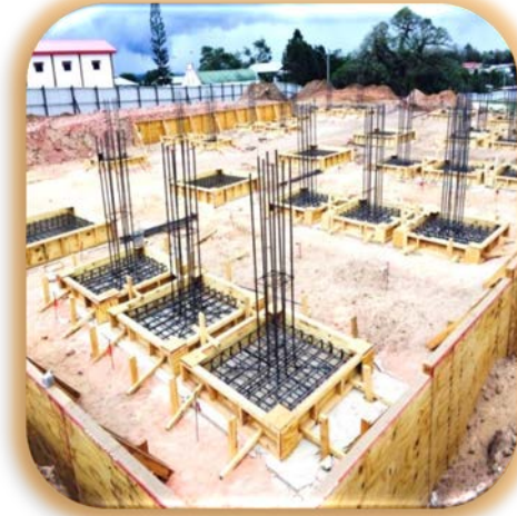
Foundation Work at Irwin Park Regional Ground
