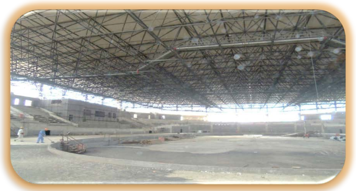
Internal view of the National Cycle Track under Construction
