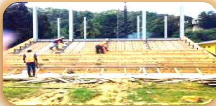
Pavilion Construction at Blanchisseuse Recreation Ground
