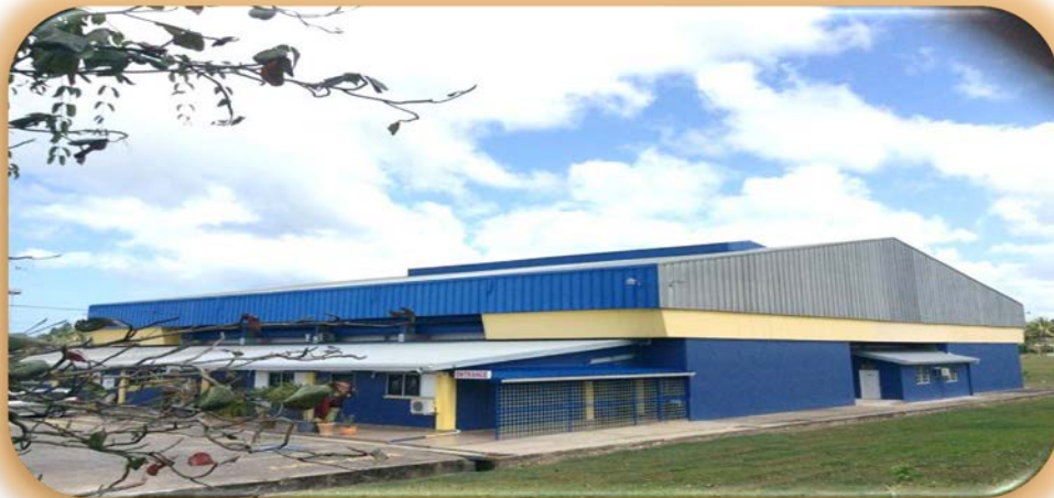
Refurbished Jack Roof at the Southern Regional Indoor Sporting Arena
