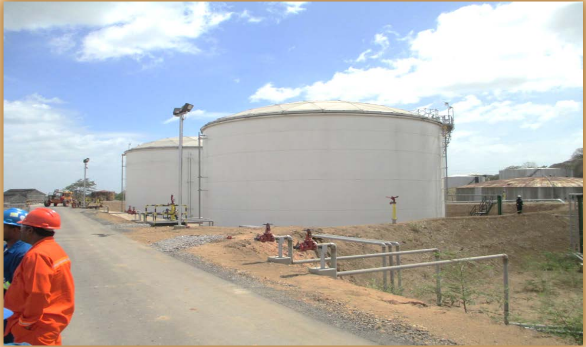
Fuel tanks at the Petrotrin West Refinery for the multi fuel Pipeline
