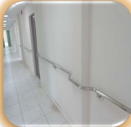
Installation of Hand rails on the corridor
