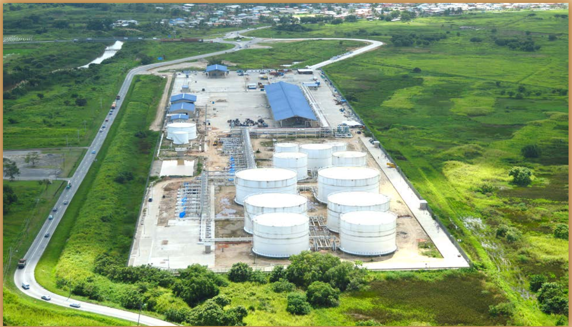
Aerial view of Multifuel Pipeline Project at Caroni
