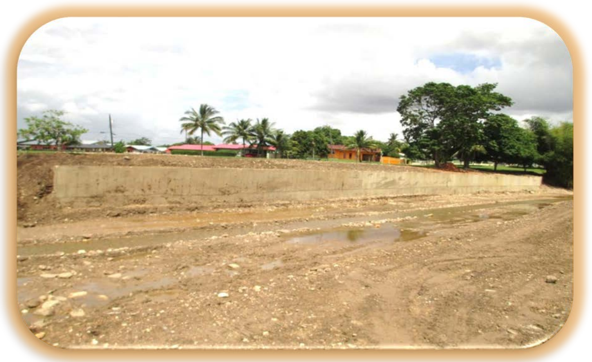
Improvement works to Arouca River Mannila Road next to the Basketball Court
