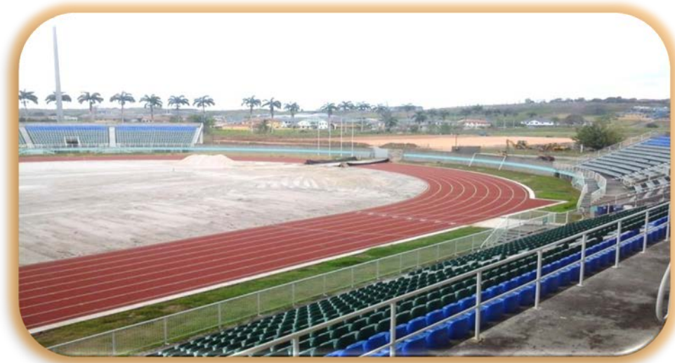
Refurbishment of Both Main & Training Field at the Mannie Ramjohn Stadium
