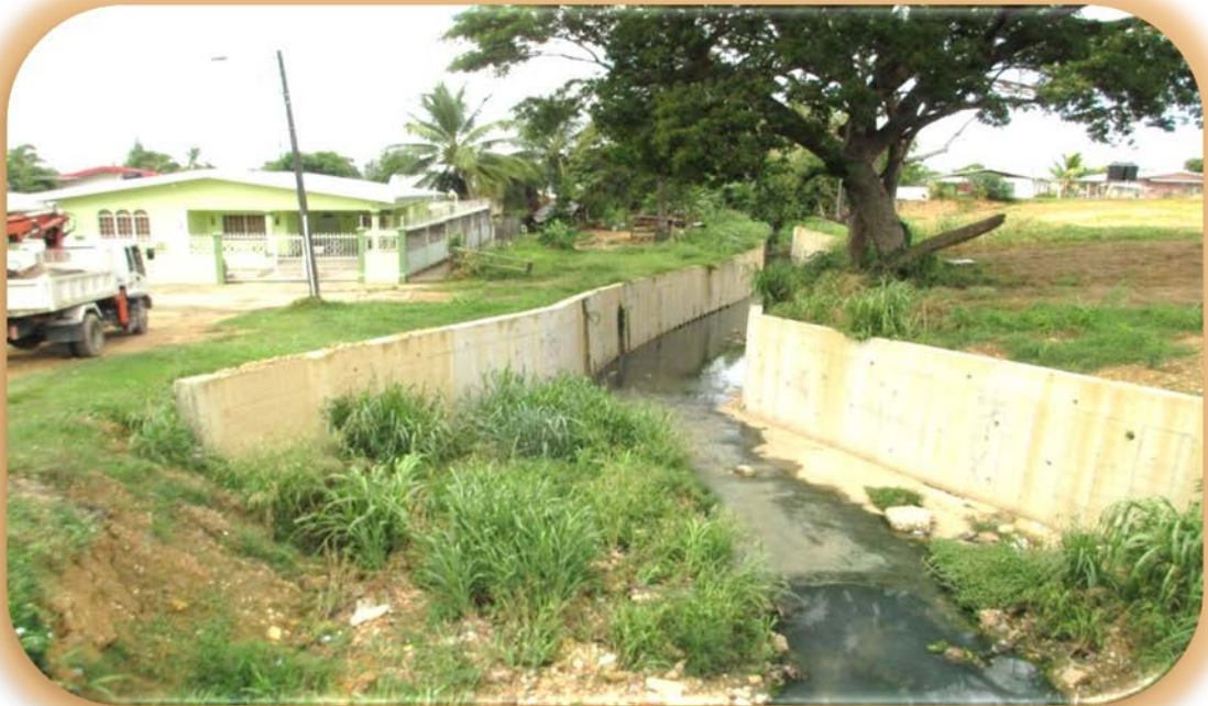
Improvement works to El Dorado Main Drain, Macoya Gardens
