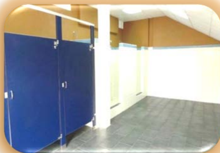
Washroom Facilities at Inverness Recreation Ground
