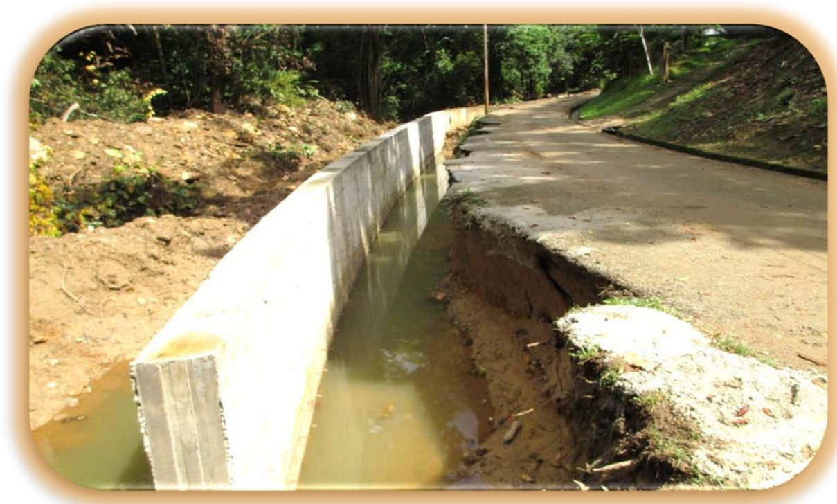
Improvement works to Tucuragua River, Caura
