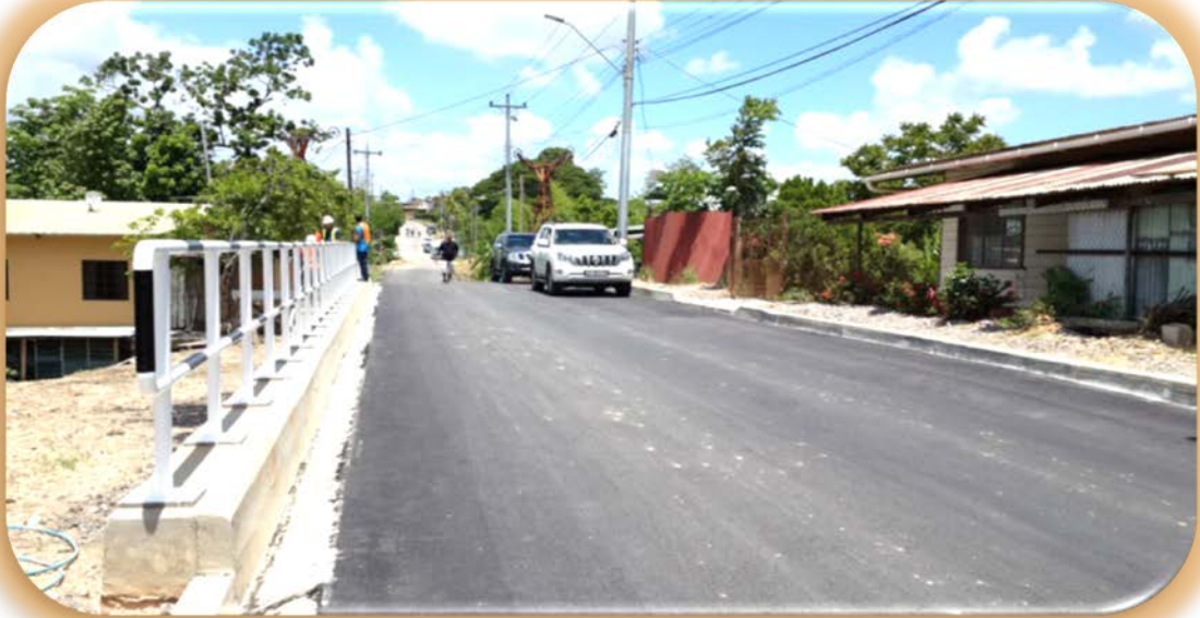
Completed Landslip repair at L36 Mayo Road
