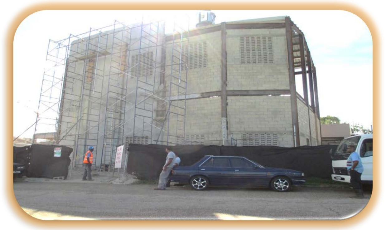
Construction of the Incinerator building at the EWMSC
