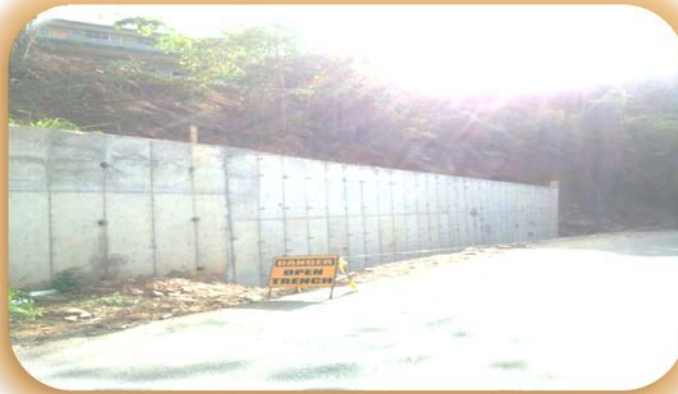
Retaining Wall at Command Row Teteron Barracks, Chaguaramas
