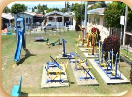
Refurbishment at El Dorado Gardens Recreation Ground
