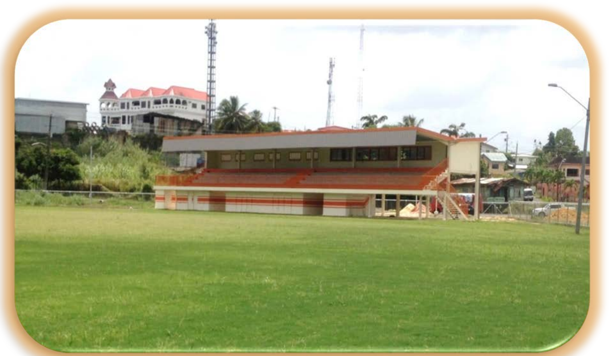
Multipurpose Pavilion at the Yolande Pompey Sub-Regional Recreation Grounds
