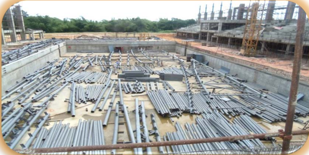
Aquatic Centre Main Pool under Construction
