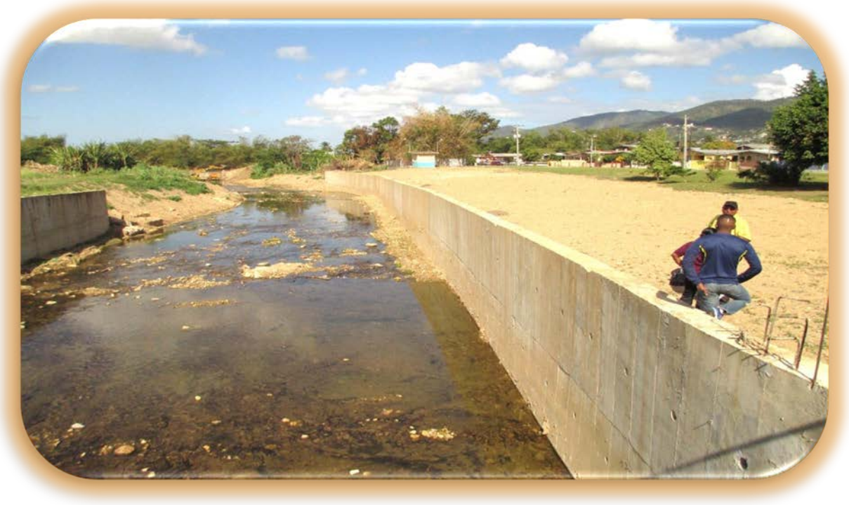
Reinforced Concrete Wall constructed on the Tacarigua River
