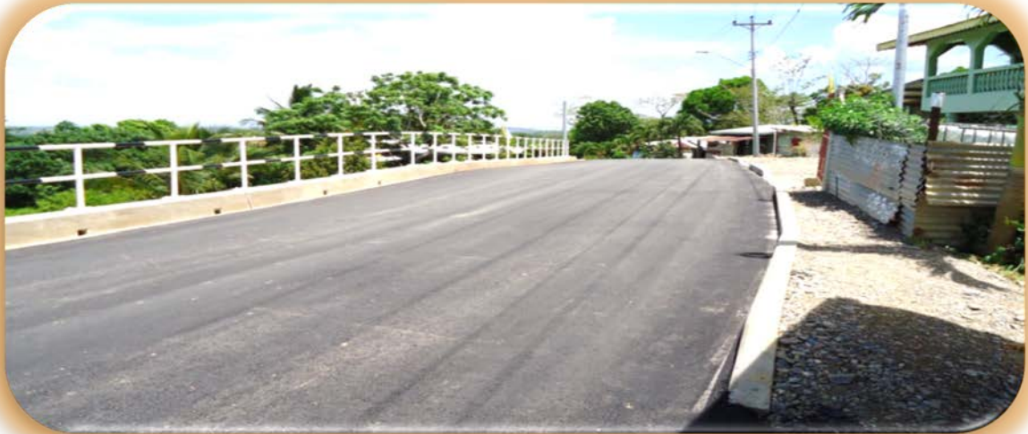
Completed Landslip repair at L38 Mayo Road
